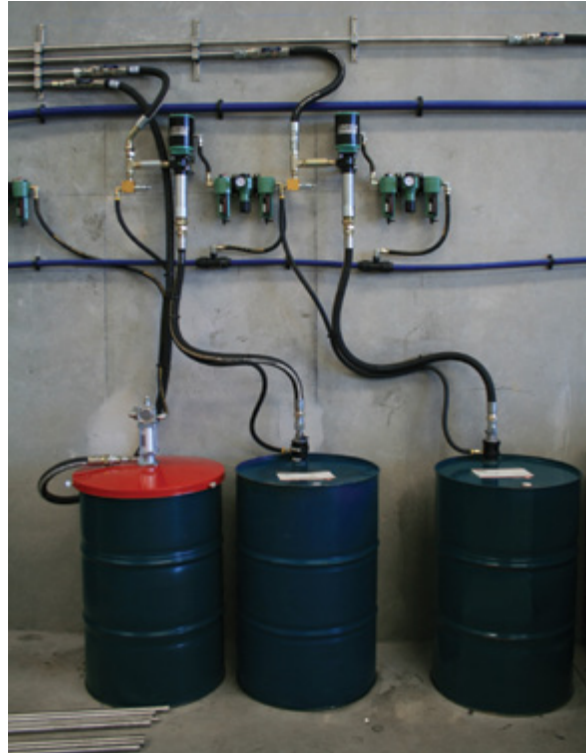
Wall mounted PMV oil pumps with remote suction
